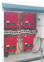
Location: Rooftop of Panasonic factory Capacity: 430 KW Inverter: 14 x GW17K-DT, 12 x GW15K-DT
